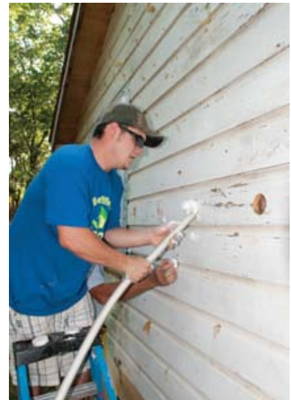
Installing RetroFoam™ through the drilled two-inch holes.
